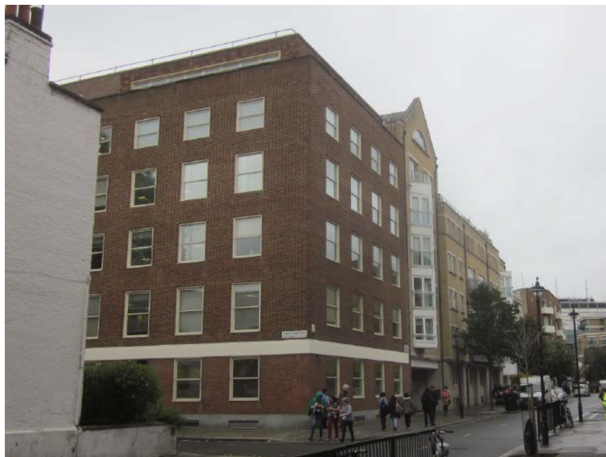
View from Regency Street showing corner of Regency St/Fynes Street
